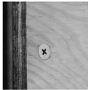
Plywood to steel or wood studs
