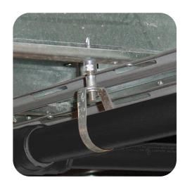
Standard Sammys technology is available for M10 metric threaded rod. Products are available for multiple substrates including wood, steel, metal deck, and concrete. UL listings and FM approvals are available.
