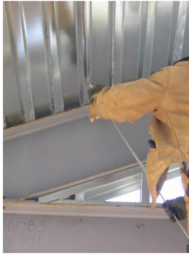
SXP Installation Ft. Bragg Construction
